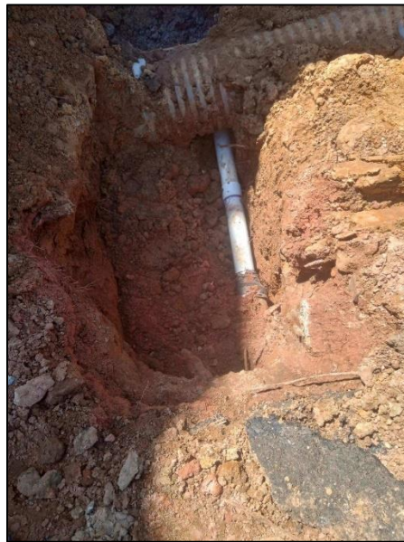
Figure 2 – New polyvinyl (PVC) pipe tie into the sewer main.
