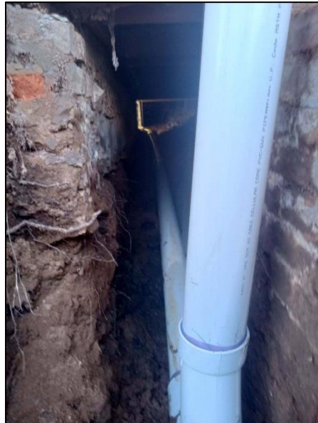
Figure 4 – Continuation of the PVC pipe depicted in Figures 2 and 3 into the crawlspace of Mr. Watts' building. Note the cleanouts as described in Mr. Slone's and Mr. Powell's emails.
