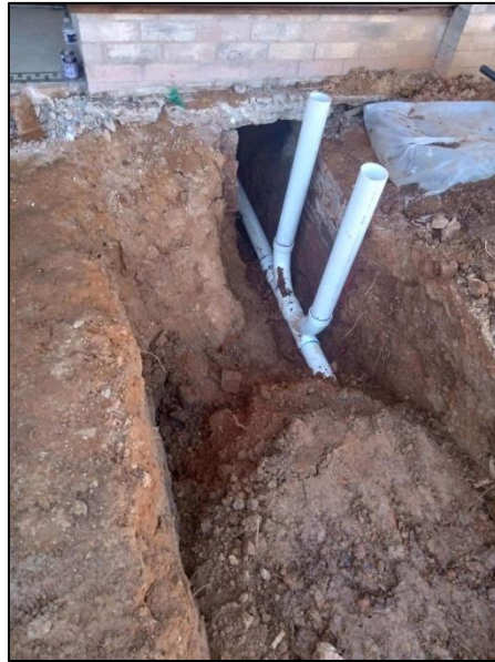
Figure 3 – Continuation of the PVC pipe depicted in Figure 2 into the crawlspace of Mr. Watts' building. Note the cleanouts as described in Mr. Slone's and Mr. Powell's emails.
